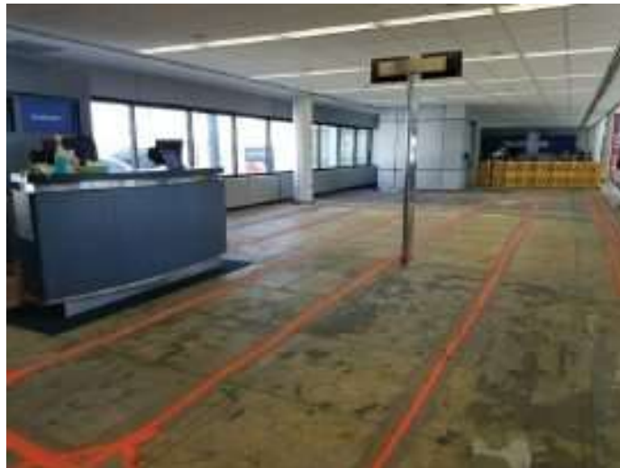
Airport managers are addressing the needs of hard-of-hearing people by installing hearing loops at departure gates, ticket and information counters, and elsewhere in their terminals.
