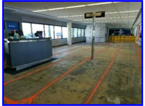
Departure gate at Rochester, NY airport being prepared for installation of phased array hearing loop
